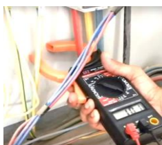
Fig. 4.19 Clamp the device around conductor
